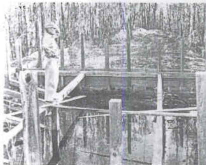
An intricate system of dikes, dams, and spillways is used to maintain water levels.
